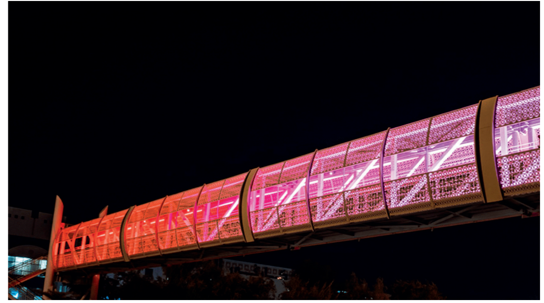
Abu Dhabi Pedestrian Bridges, UAE
